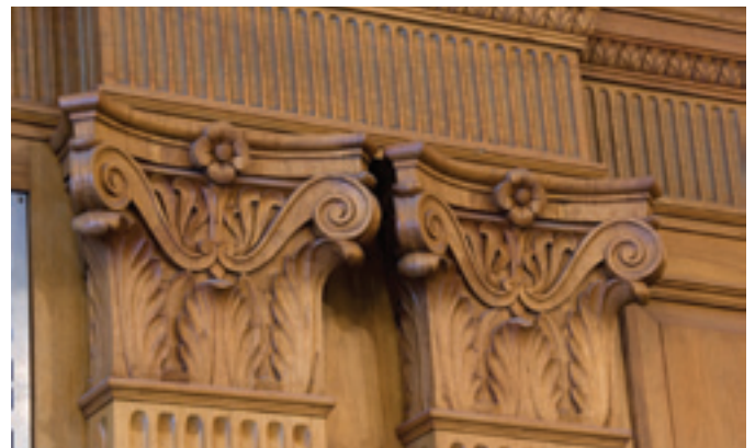
Two photos above: intricately carved design above the doors (left) and detail of the crown moldings on top of hand carved walnut pilasters. The wood paneling is 10 feet in height and outlines the perimeter of the centrally located reception room.
