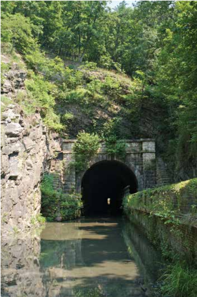
The Paw Paw Tunnel, an engineering marvel constructed of more than six million bricks, runs three-quarters of a mile. Tunnel engineers estimated construction would take 2 years, but ultimately took 14 years to build. PHOTO BY LANCE BELL
