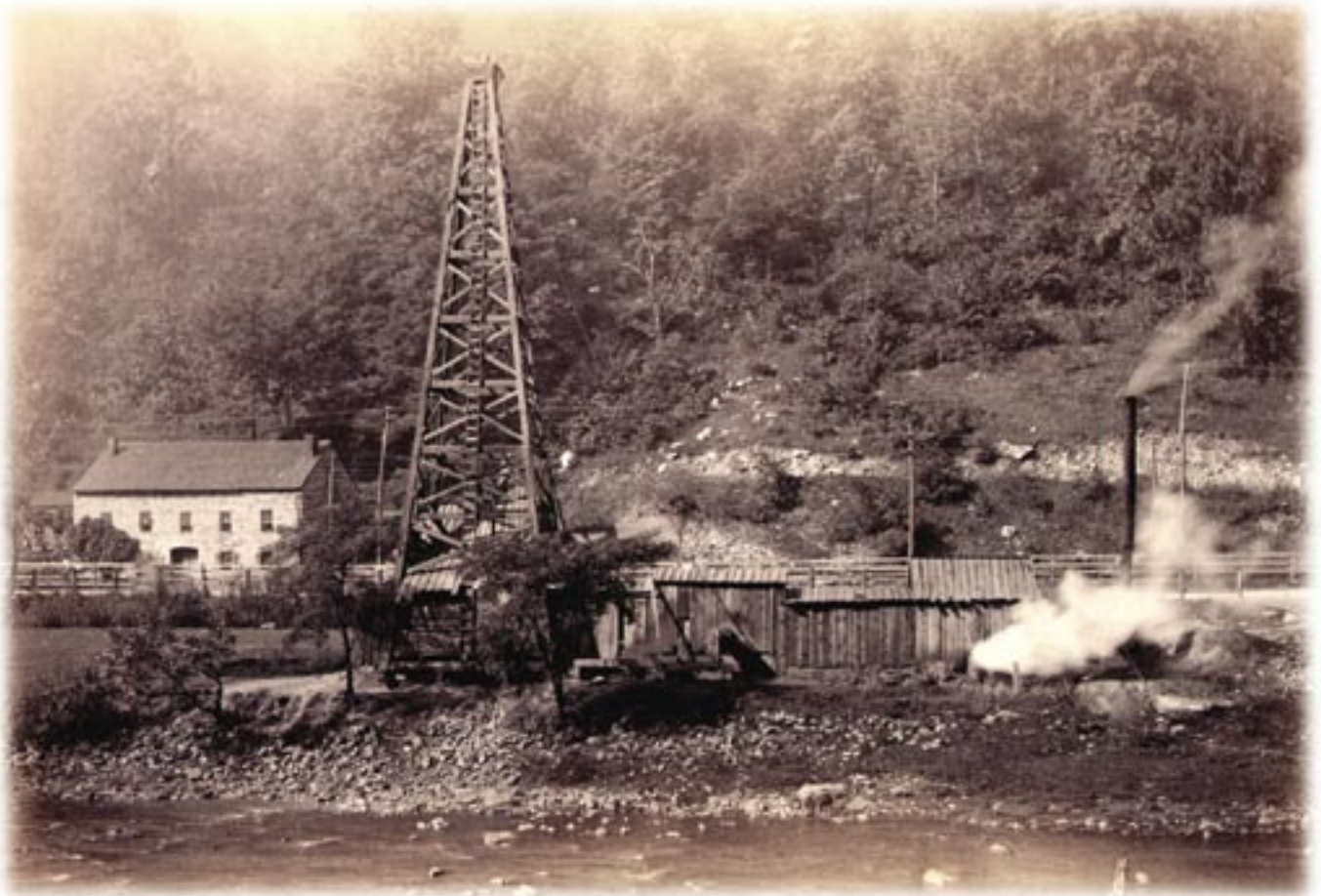
Oil well sank in the Narrows (near Fruit Bowl). Well was sunk in July 1903 and by September was producing three barrels of oil per day ($100. per annum for any oil produced). Abandoned shortly afterwards. Owned by the Tuscarora Oil Co., Incorp. in West Virginia, part of Narrows land leased to Atlantic Refining Co.
